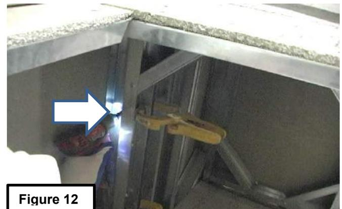
**NOTICE** Use of non-galvanized screws can rust and fail. Screw failure is dangerous and should be avoided by using properly coated screws.
